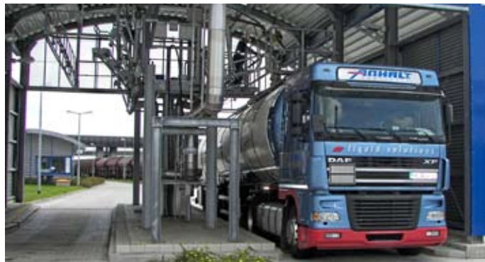
Modern tanker loading facility at SKW Piesteritz
